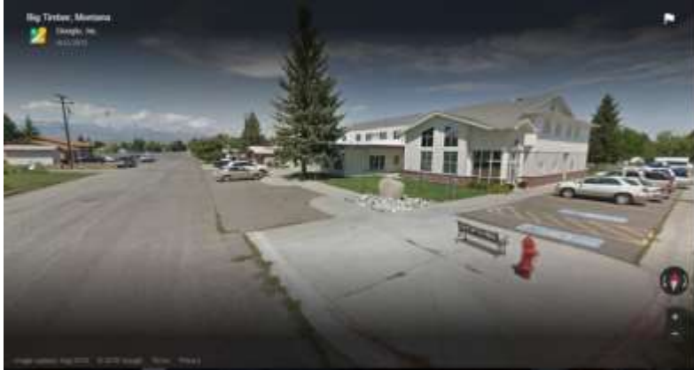
Entrance to the Boulder Meadows Assisted Living Facility (Google Maps)
