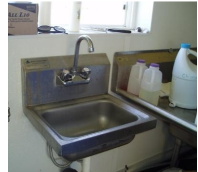
Self-closing doors and separate hand-washing sinks reduce the risk of contamination.
